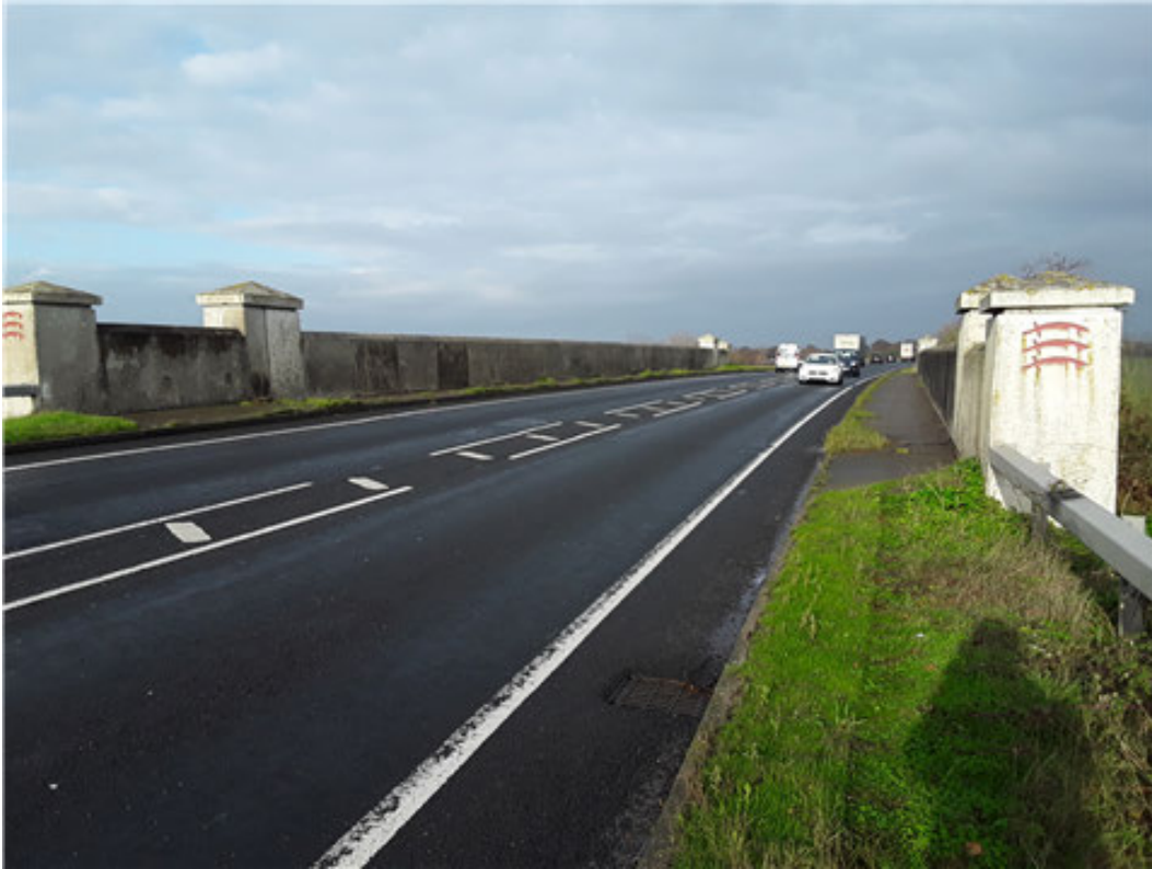
South Topside (looking north) South Topside
