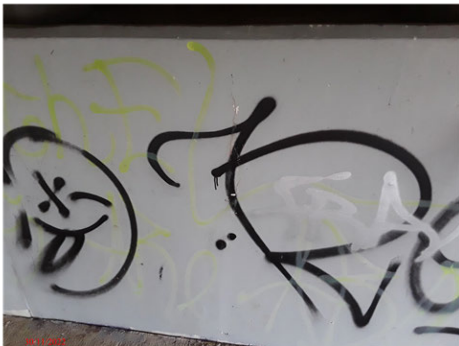
Span 1 - South West Abutment Vertical hairline crack
