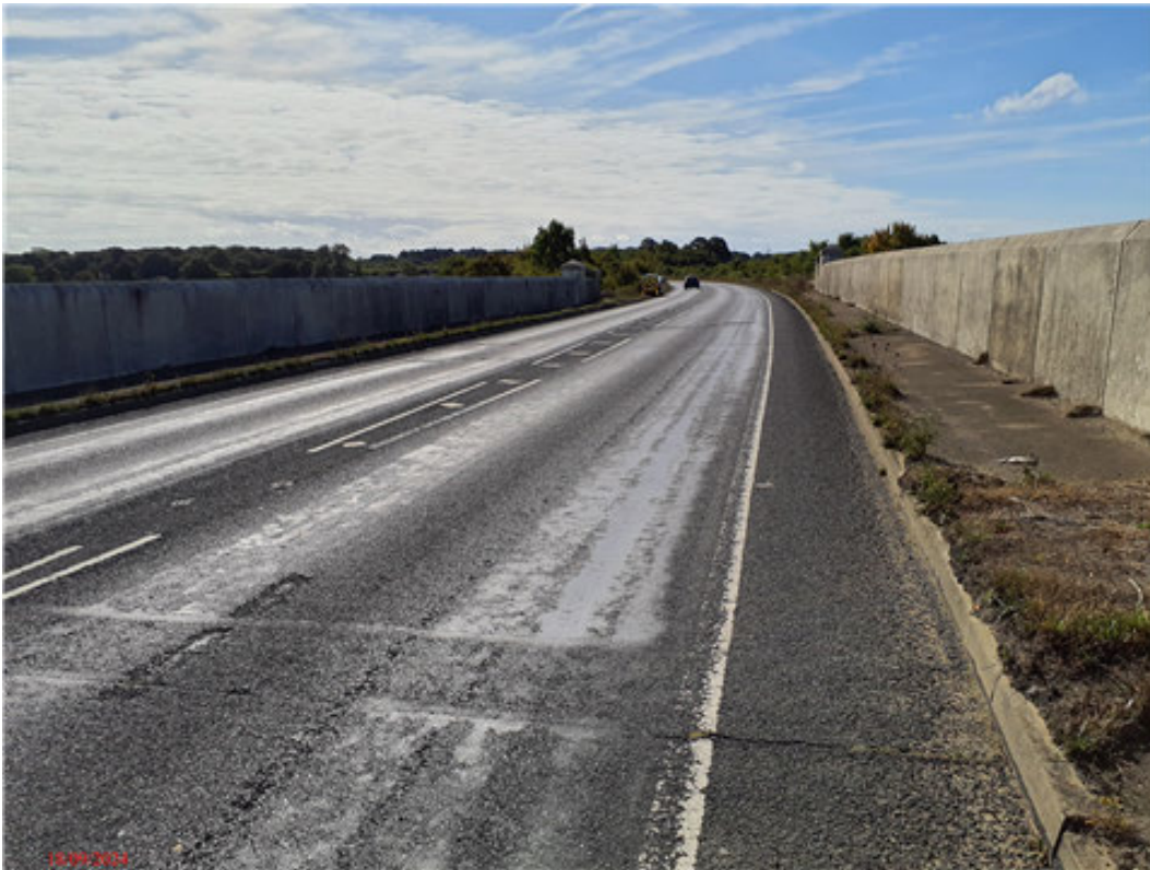
General Photograph 1 General view looking south along the top of bridge.
