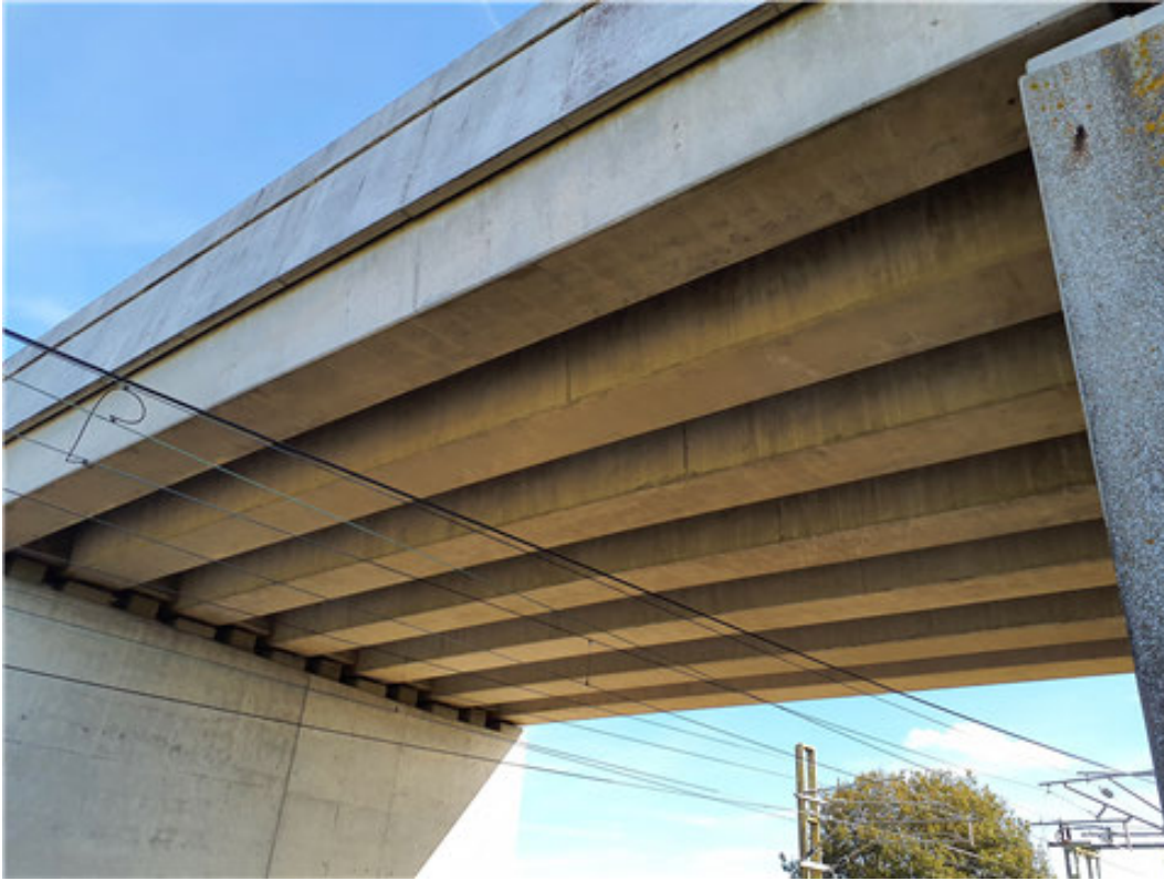
General Photograph 2 General view of the deck soffit of span 2.
