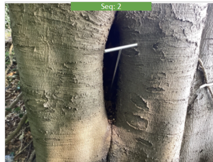
30/06/2025: Trunk - Trunk cavity
