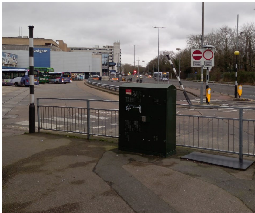
RSA 3-4 Image 4 – Damaged pole and globes at crossing
