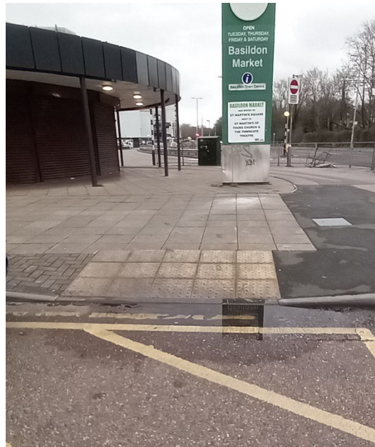
RSA 3-4 Image 4 -standing water at crossing point
