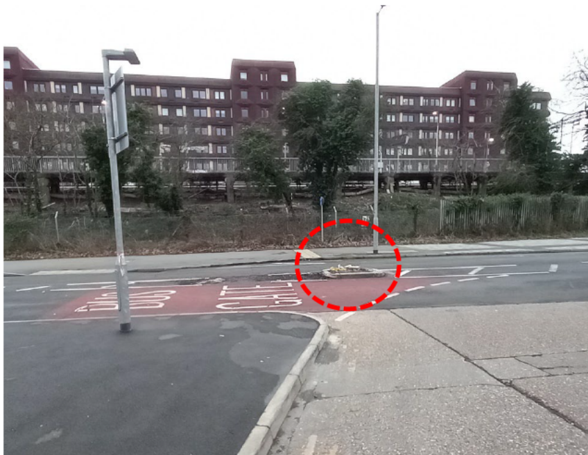
RSA 3-4 Image 5 – Damaged/removed traffic sign assembly on Southernhay at Bus Gate.
